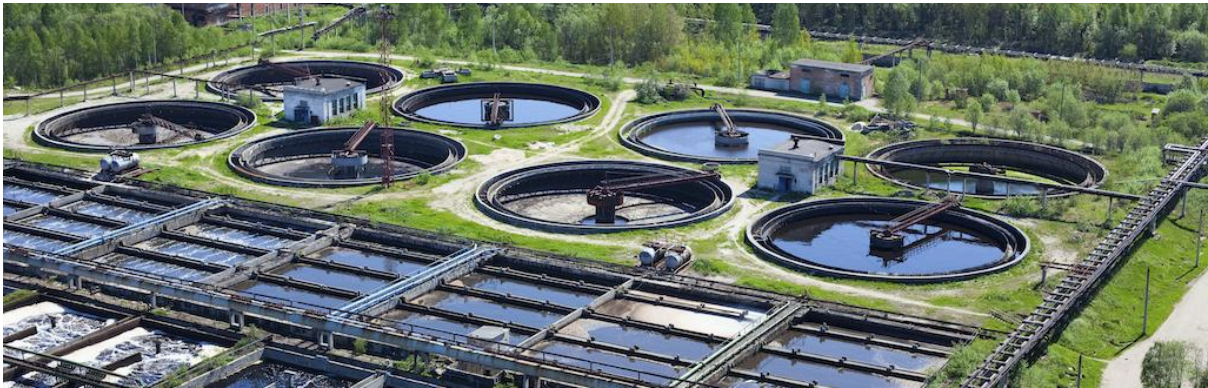
A wastewater treatment plant.
