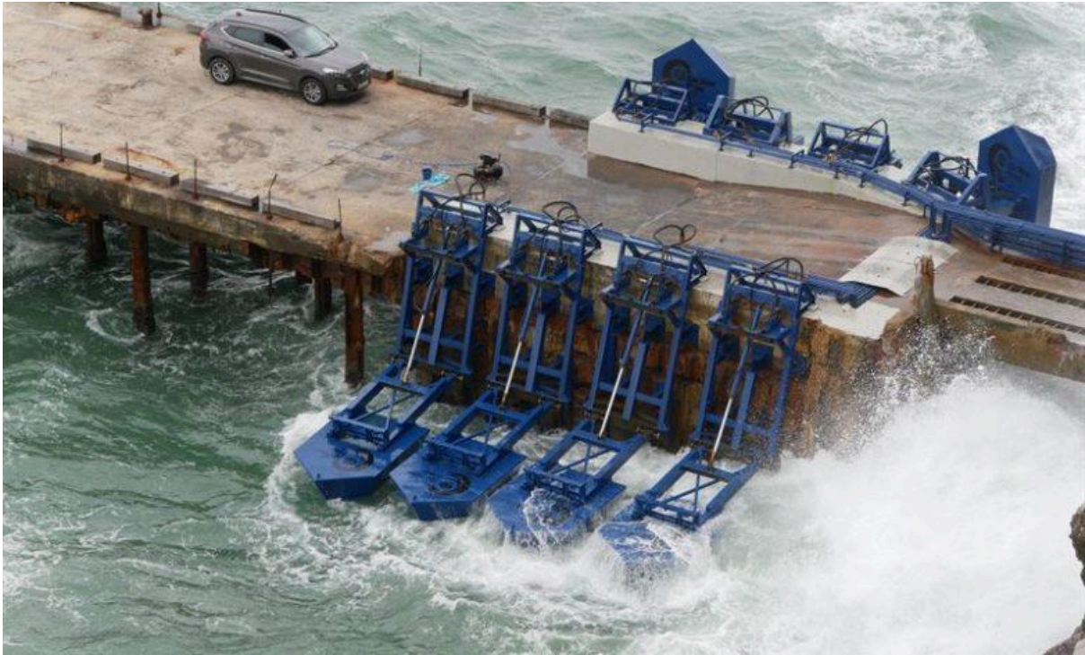
A picture from a wave power plant.
